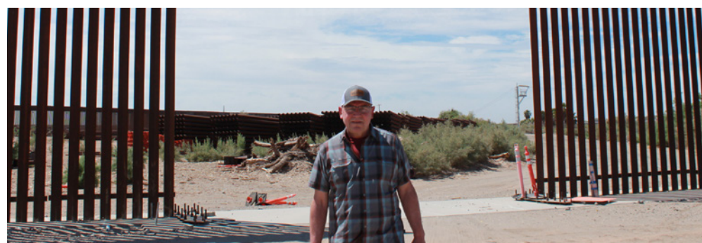
Congressman Tiffany stands in between a gap in our southern border wall where already bought and paid for border wall materials lie behind him, rusting in the Arizona sun, due to President Biden's Executive Order to halt all border wall construction.
